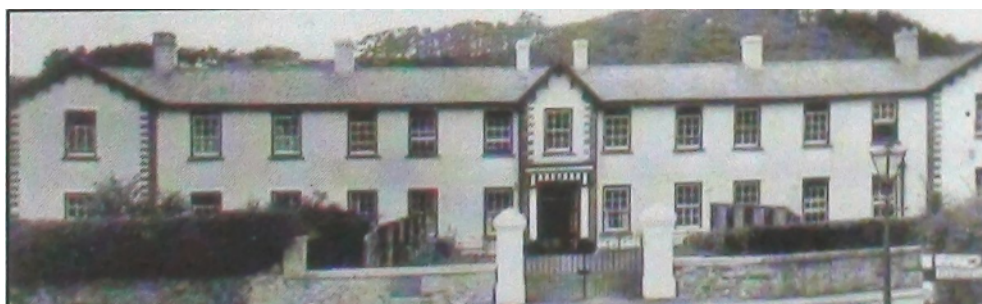
The Union Workhouse, Machynlleth which later became the King Edward VII Hospital, known as the Chest Hospital.
